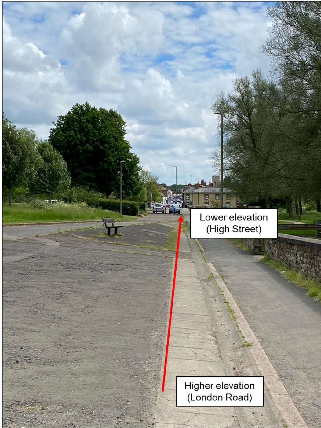
Figure 1-3 - Evidence of drop in elevation from London Road (north) to the High Street (south) that might encourage conveyance of surface water runoff to the High Street located in local low point.
