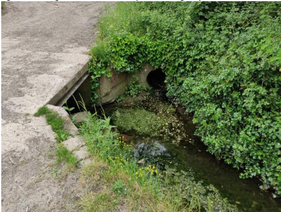
Figure 4: Convergence of watercourses upstream of highway
