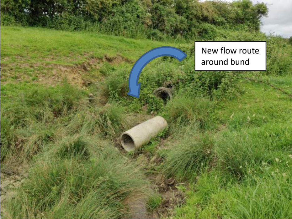
Figure 4: Bund 2 (Failed) - with new flow route
