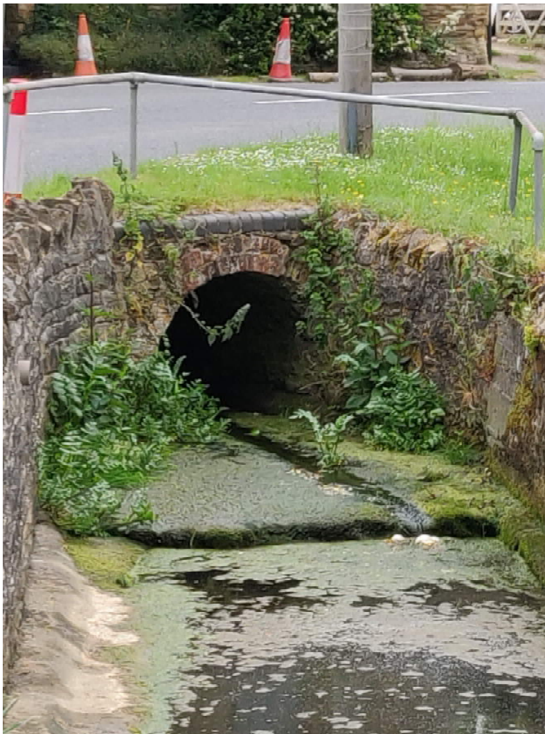
Figure 2 Watercourse looking upstream away Tathall End
