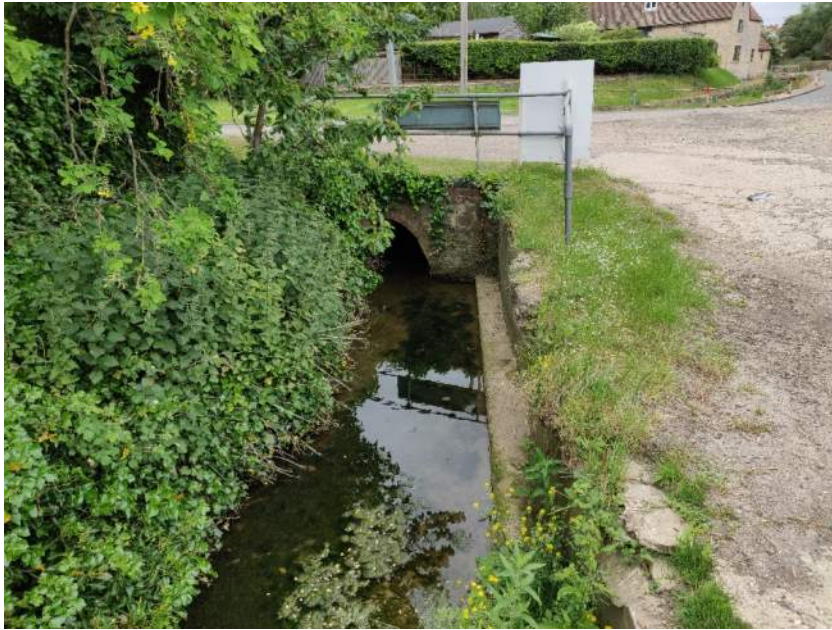
Figure 3: Watercourse looking downstream towards Tathall End
