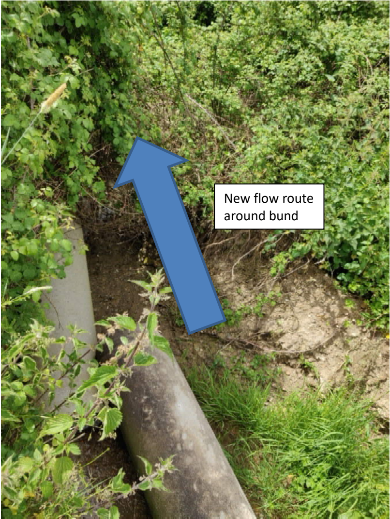
Figure 4: Bund 2 (Failed) - with new flow route
