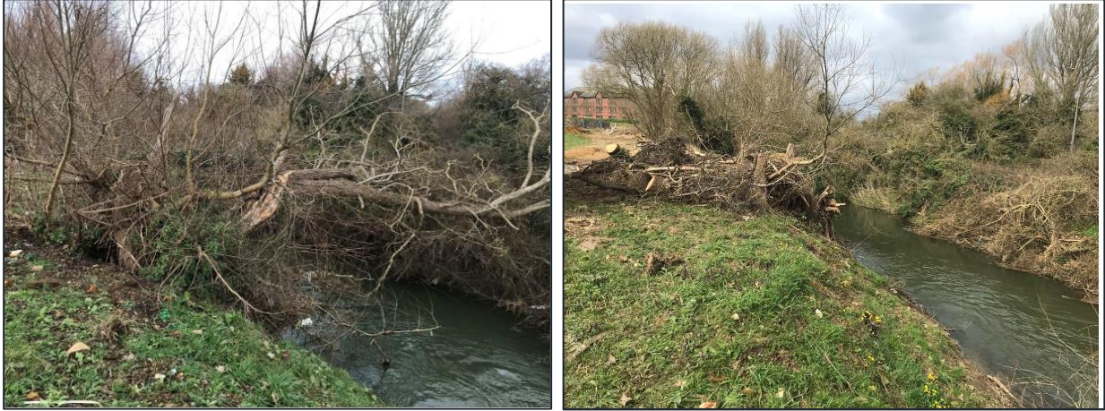
Figure 1-6 – Pre and post maintenance photos upstream of Watling Street Bridge
