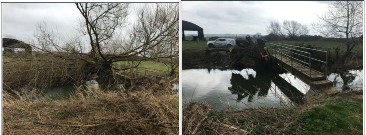
Figure 1-7 – Pre and post maintenance photos of Waterhall Park at the pedestrian bridge on Mill Road
