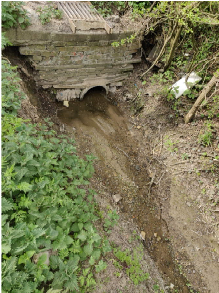
Figure 6: Silted Culvert on High Street
