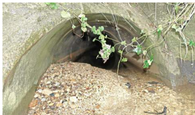
High St East Adjacent to site Sand in drainage tunnel to west (site)
