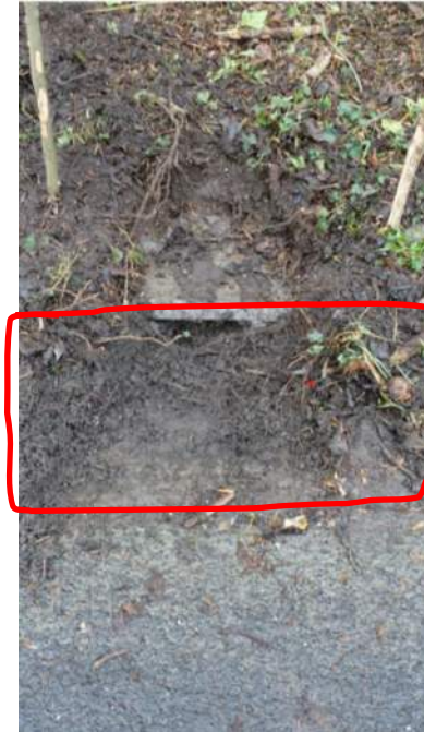
High St West Recovered Drain Road Loss to overgrown vegetation
