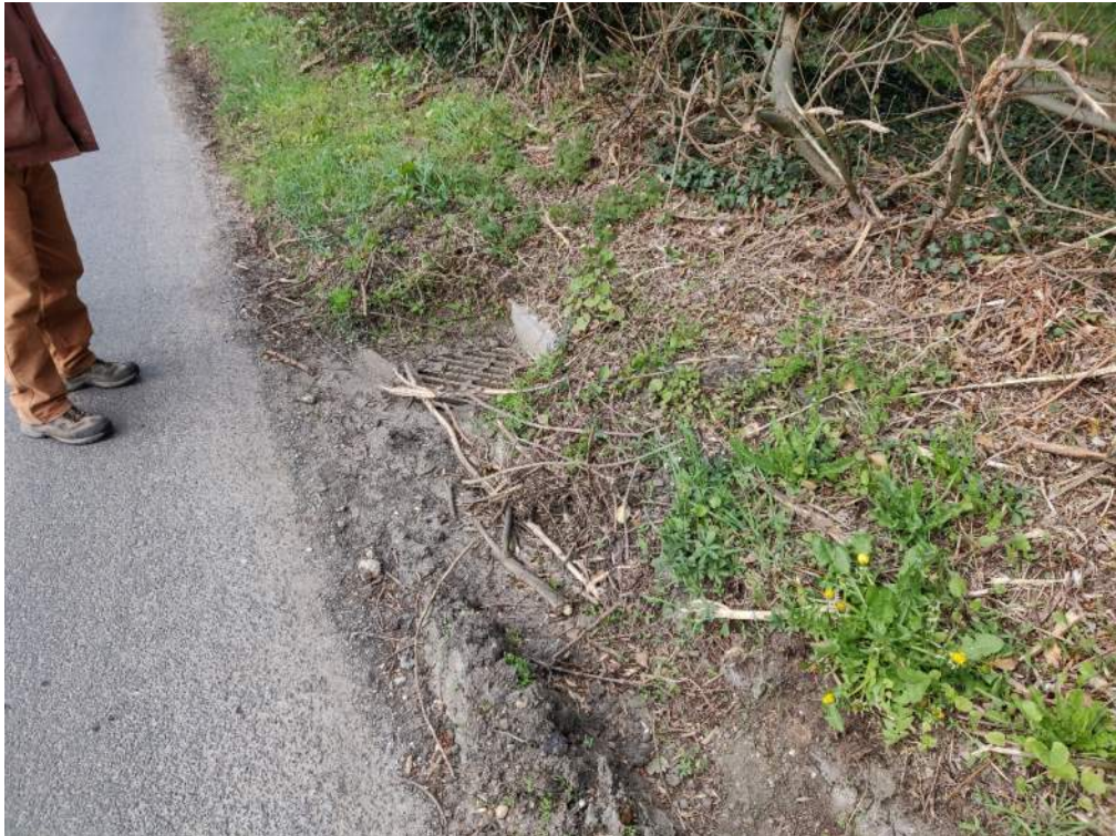
Figure 6: Silted Culvert on High Street
