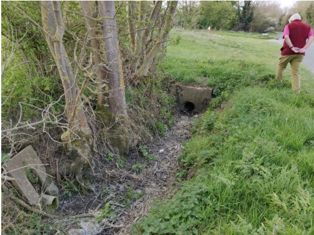
Figure 3: Culvert on High Street under Gun Lane
