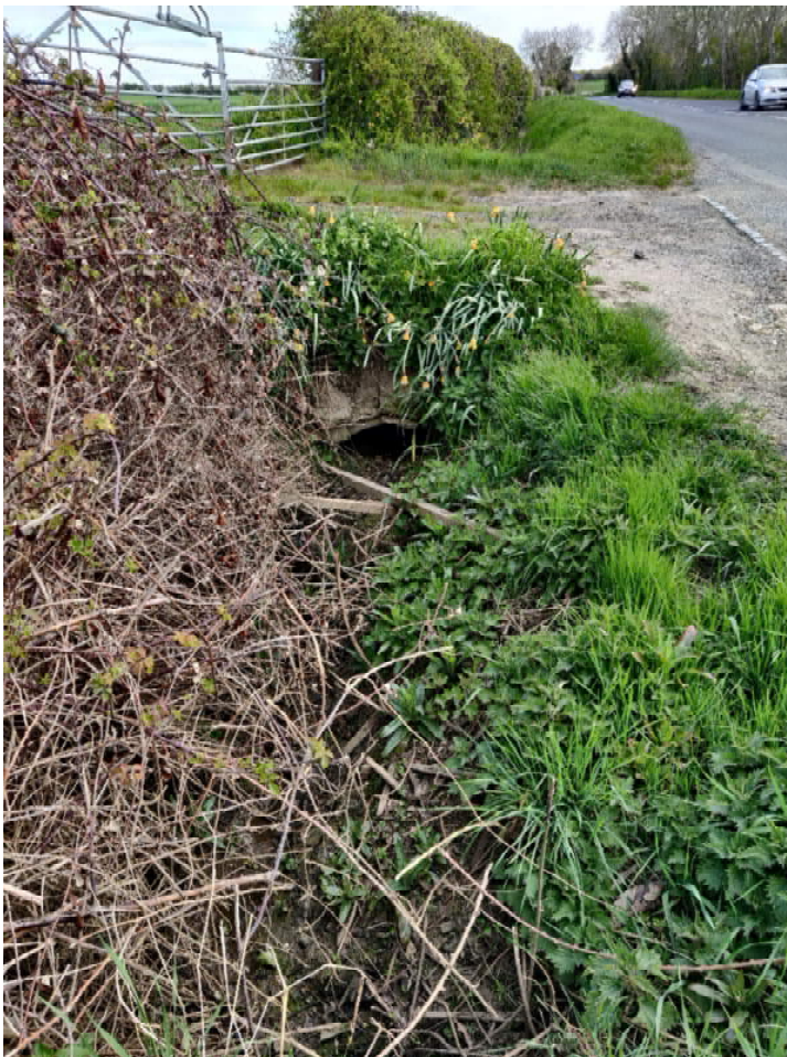
Figure 4: Culvert on west side of High Street near Gun Lane
