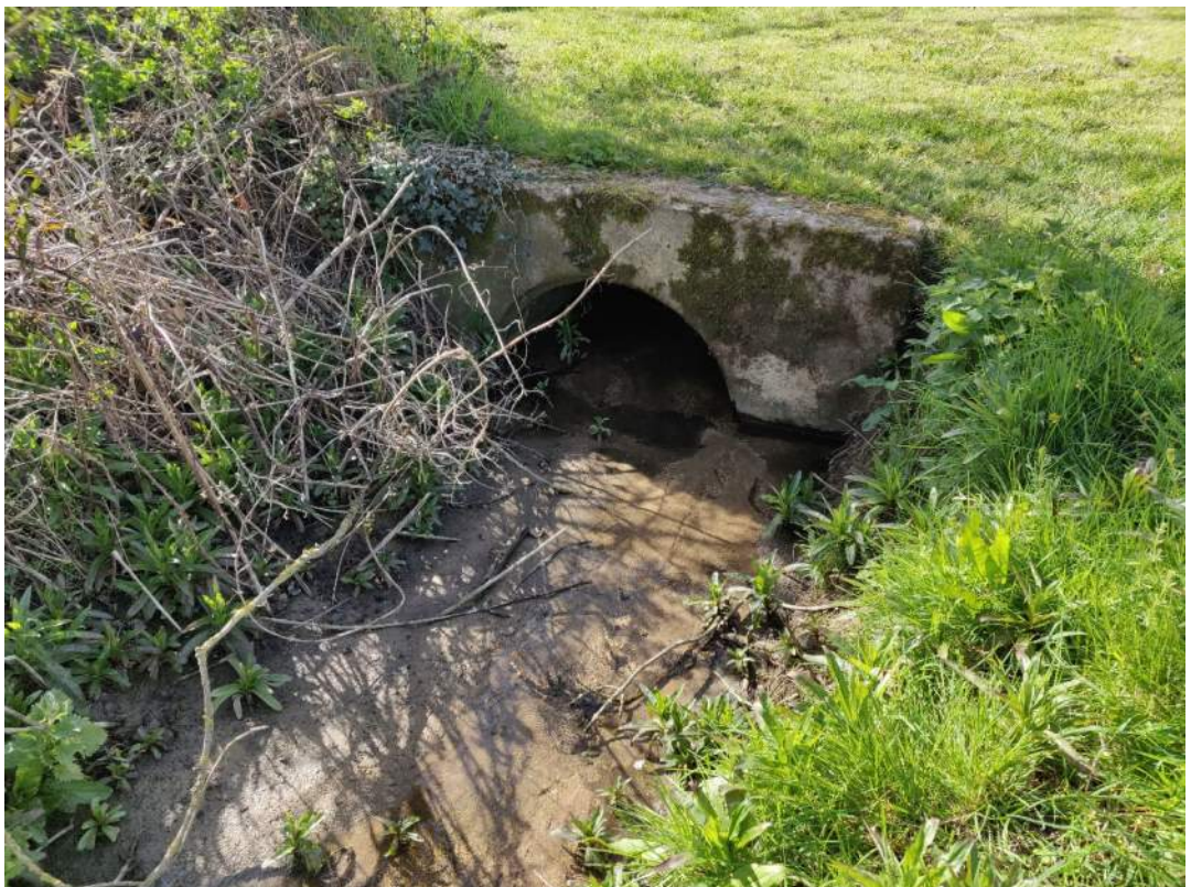
Figure 10: High Street Ditch partially blocked with Silt
