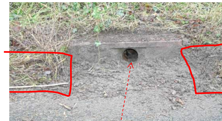
High St East, Cleared kerb drain Vegetation overgrown
