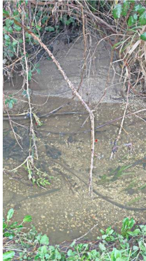
High St East Sand in ditch
