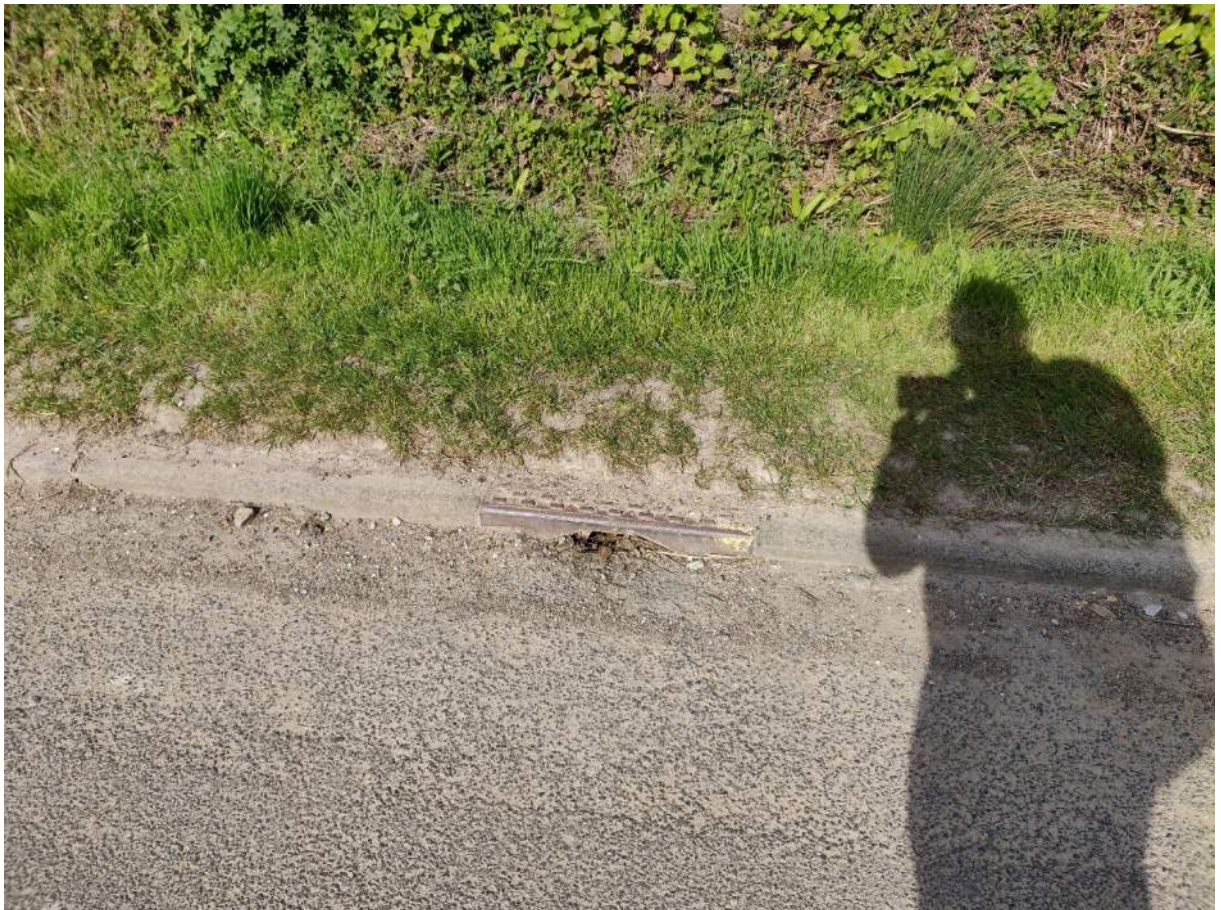
Figure 8: High Street Road Drainage
