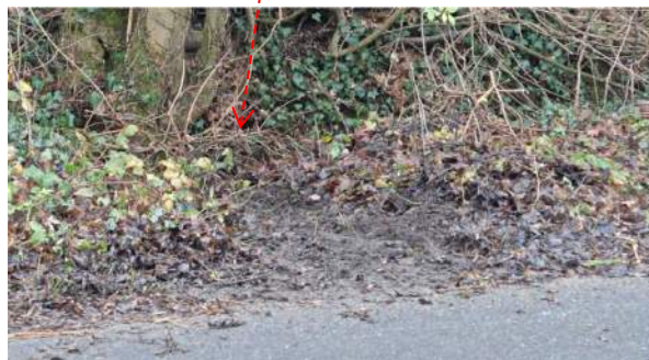
High St East Cleared Run off
