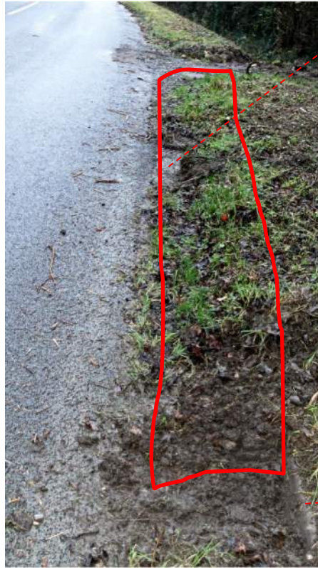
High St West Recovered Drain Recovered Kerbside Road Loss to overgrown vegetation
