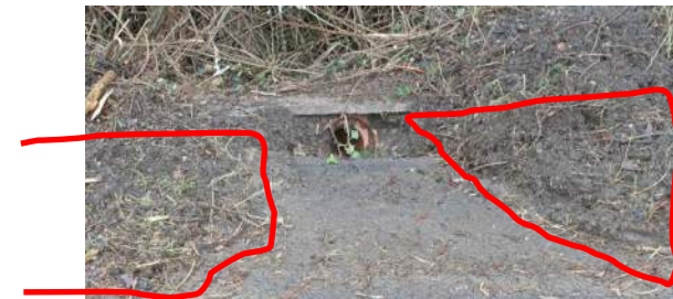
High St West Recovered Drain Road Loss to overgrown vegetation
