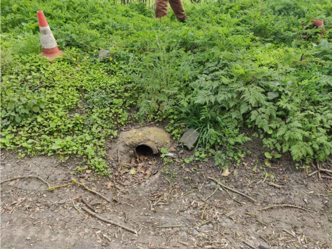
Figure 1: Gun Lane Road Drainage – kept clear by residents
