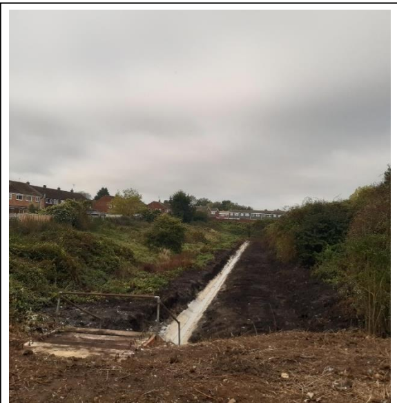
Figure 3: Conveyance infrastructure near Angus Drive
