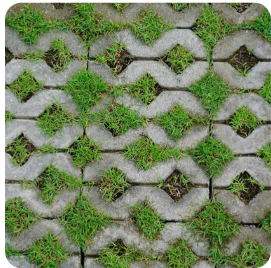
Grasscrete is an option to protect a grass verge from vehicles
