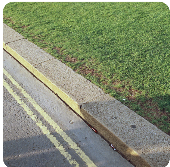
Granite kerb in CMK with double yellow lines
