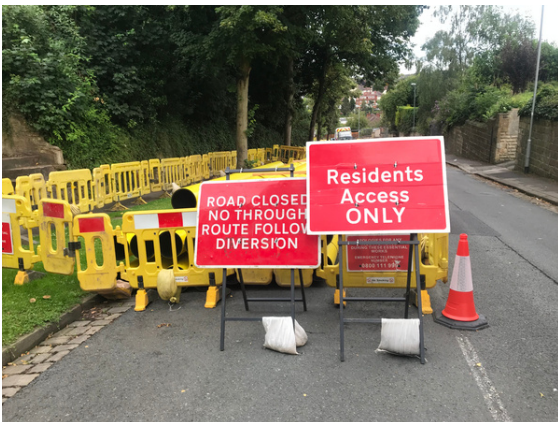
Streetworks taking place to install utilities pipes in the verge.
