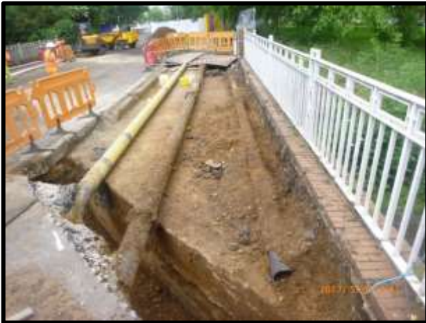
Removal of an empty pipe GAS
