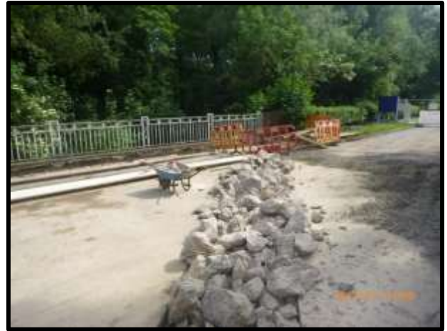
Back of the abutment excavated in preparation for waterproofing
