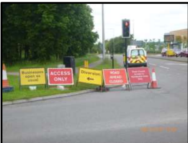
5 No. Signs at Newport Road near Saxon Street V7 junction
