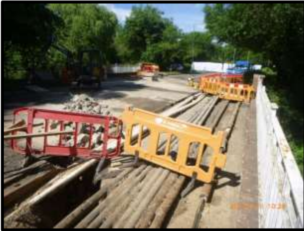
Concrete bridge deck and Statutory Undertakers Apparatus exposed
