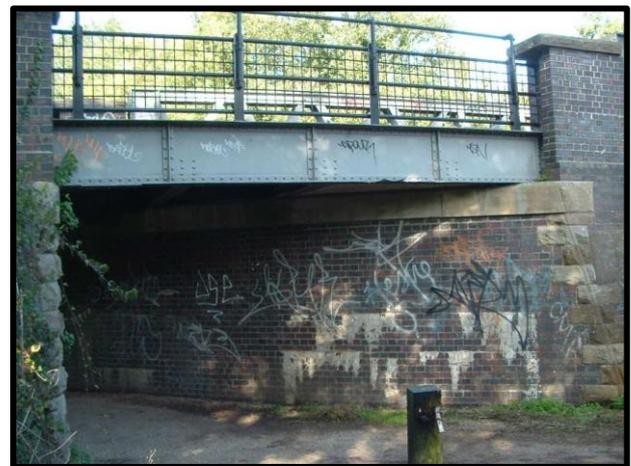
South Elevation of the plate girder bridge
