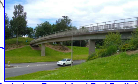
Eaglestone Roundabout East Footbridge MKC No. 86375A
