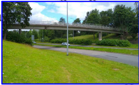
Eaglestone Roundabout North Footbridge MKC No. 86375D
