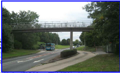
Greenleys - Hodge Lea Footbridge MKC No. 81392
