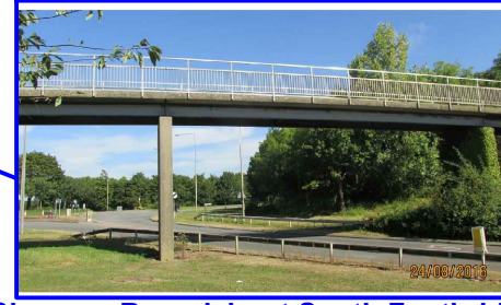
Simpson Roundabout South Footbridge MKC No. 87361
