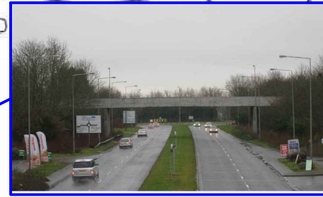
Porthleven Place Footbridge MKC No. 86388
