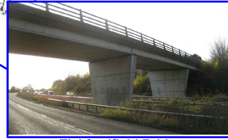
Tickfordfield Bridge MKC No. 89432
