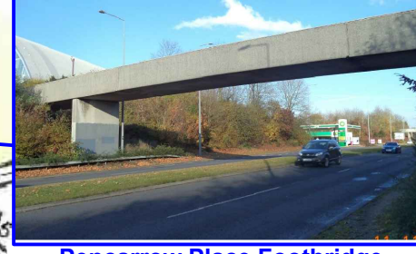
Pencarrow Place Footbridge MKC No. 85388A
