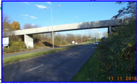
Cranesbill Place Footbridge MKC No. 85392B
