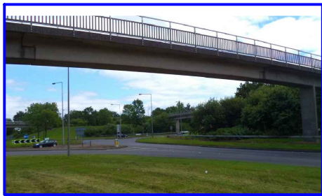
Eaglestone Roundabout West Footbridge MKC No. 86375C
