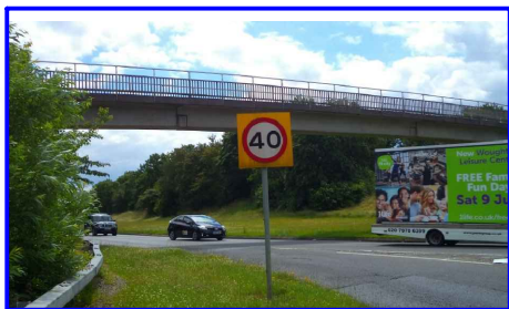
Eaglestone Roundabout South Footbridge MKC No. 86375B
