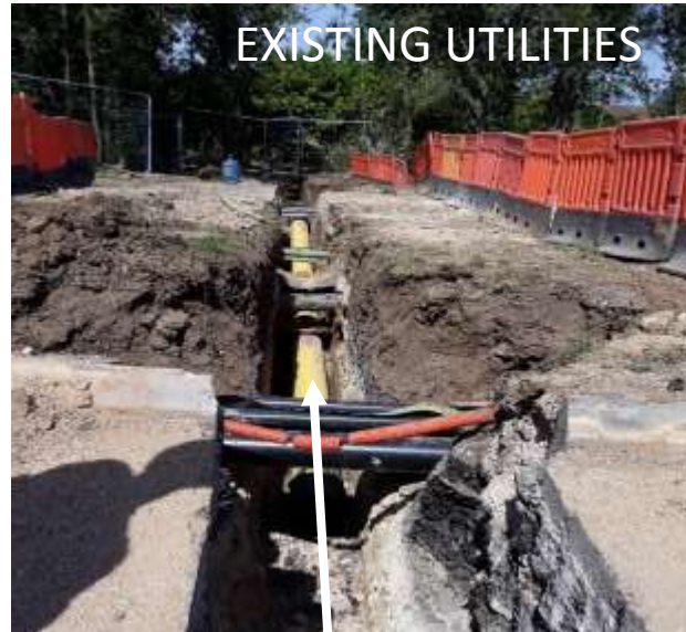
New Gas diversion pipe being laid (yellow duct)
