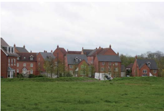
Housing facing the eastern edge of the site along Cranborne Avenue. The slope of the site is evident
