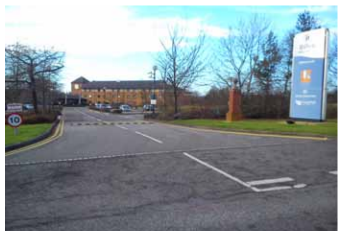
The Hilton Hotel viewed from Timbold Drive
