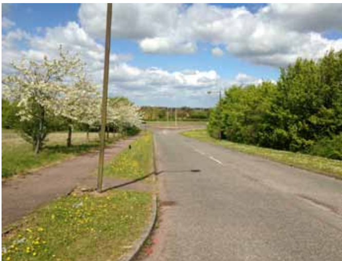
Durgate providing access off the H8 and connecting with Tmbold Drive
