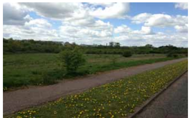
Site A which is largely featureless slopes gently away from Timbold Drive
