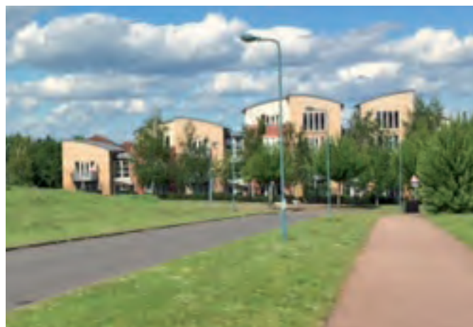
3 and 4 storey apartments addressing the corner of Coulson Avenue and Oldham Rise which overlooks the sites.
