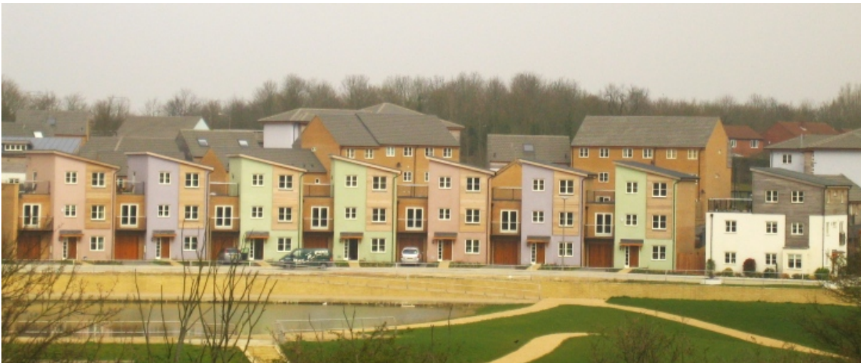
Picture 3 Housing at Ashland
