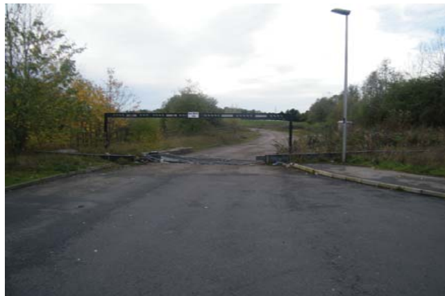
The northern entrance to the site off Wansford Avenue
