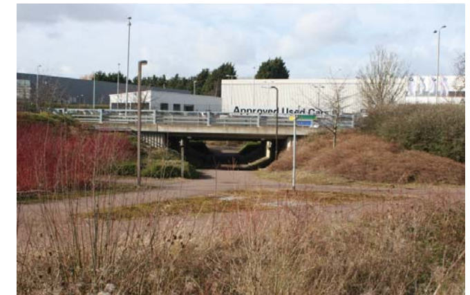
Existing redway underpass connecting site to Northfield
