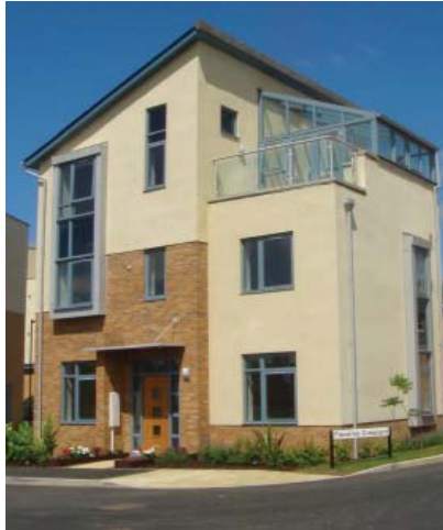
The uniform palette of materials and contemporary design has helped create a strong character for this development
