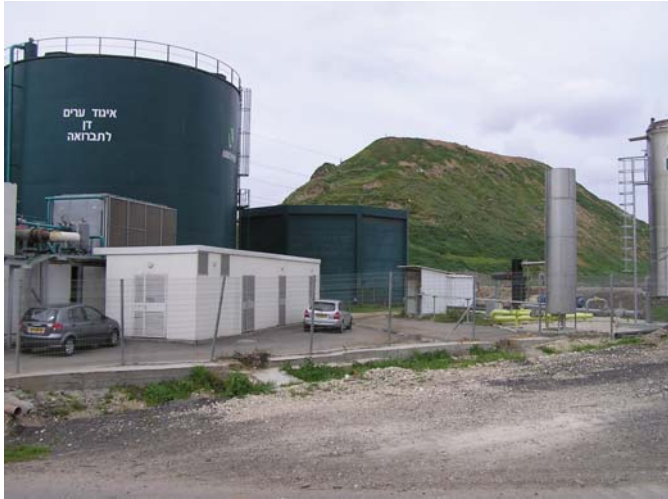
Anaerobic Digester in Tel Aviv
