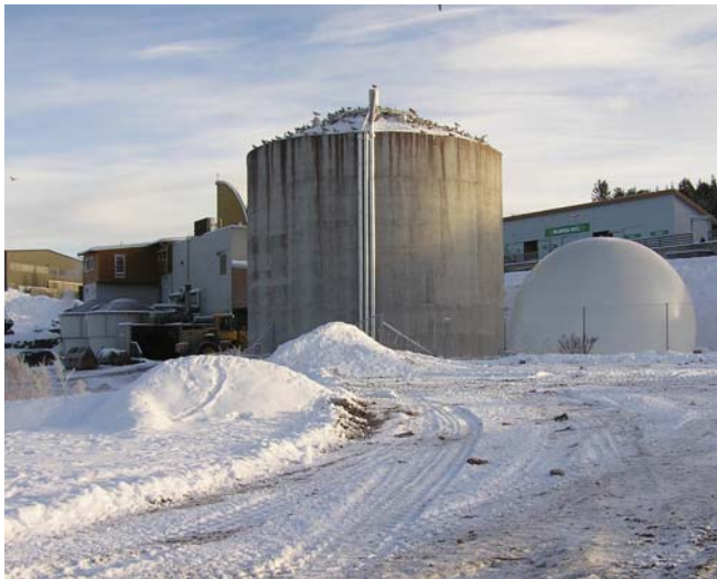
Anaerobic Digestion facility, Lillehammer
