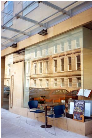
Shopfront and façade improvements will improve the retailing environment along Queensway
