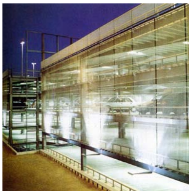
Attractive multi-storey car parking
