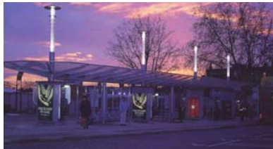
Quality bus stops provide shelter from the elements – improving user experience
