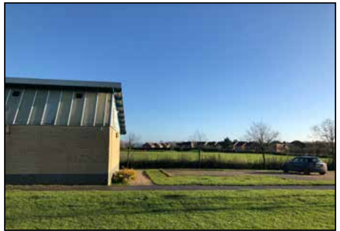
Kents Hill Sport Pavilion positioned on opposite side of playing field to the site
