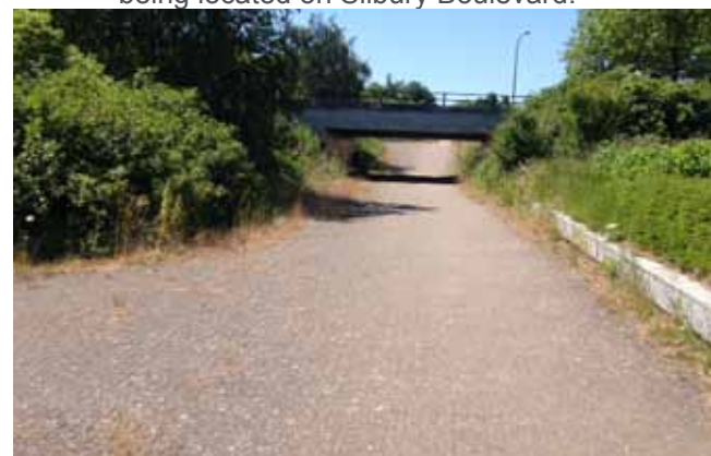
Redway and existing underpass underneath Skeldon Gate which runs alongside the southern edge of the development sites
