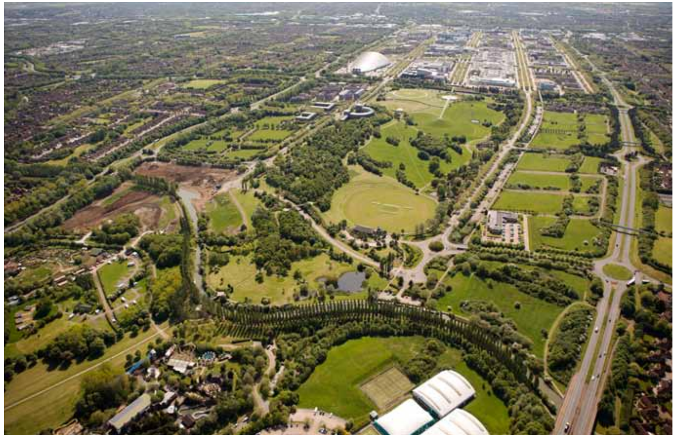
Campbell Park Northside with adjacency to the city centre, Campbell Park, the Grand Union Canal and Newlands
