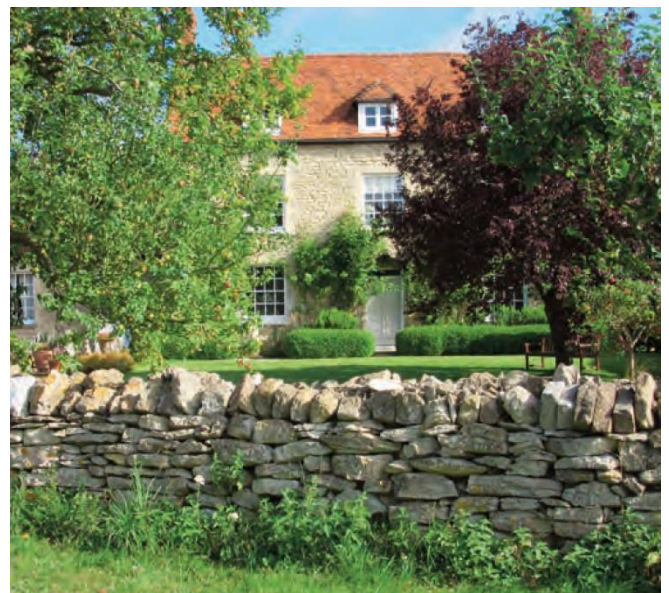
A vernacular scene at Sherington with local tile and stone. Note the open joint (mortar free) traditionally made boundary wall.
