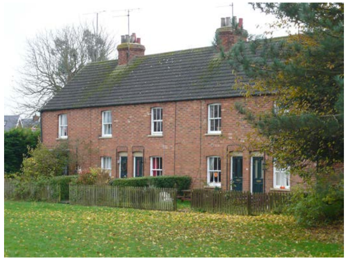
16. Victorian farmworkers' cottages on The Green
