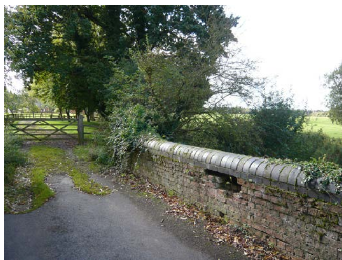
40. Victorian bridge to Equestrian Centre
