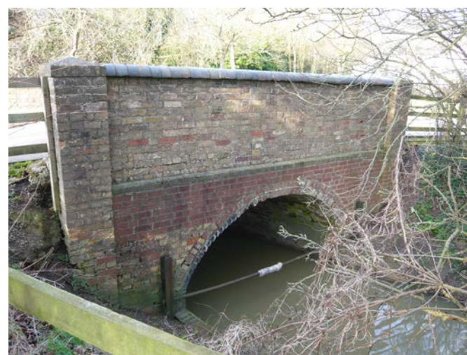
30. Victorian bridge on Leys Road
