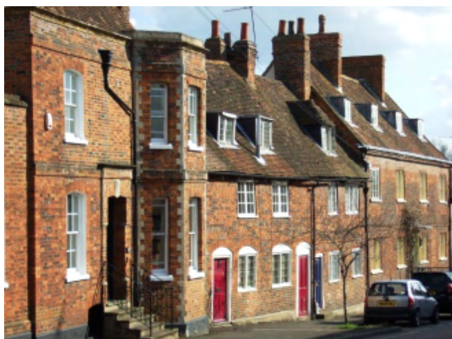
Picture 11 Houses on Silver Street
