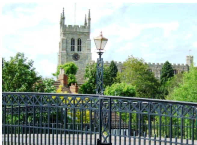
Picture 16 Tickford Bridge and Church
