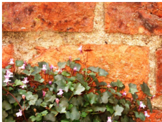
Picture 27 Lime pointing (minerals in the lime will encourage plants to grow; creepers such as ivy should be discouraged, however)
