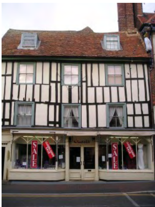
Picture 26 Timber framing in High Street
