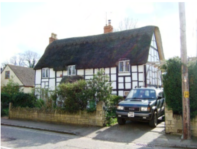
Picture 14 Timber Framed House, Caldecote Street
