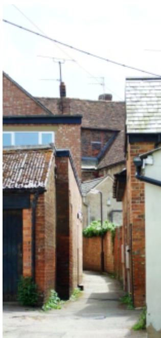
Picture 5 A narrow passage through cramped rear yards
