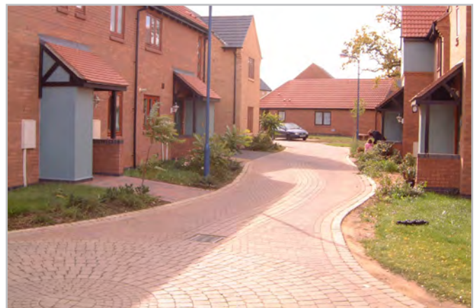
Level surface street too narrow, with poorly defined and overly sinuous edges resulting in vehicles overrunning the carriageway and being unable to pass through when cars are parked in the street.
