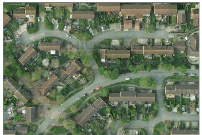
Florin Close, Leopard Drive, Noble Close in Pennyland - buildings positioned to capture solar gain
