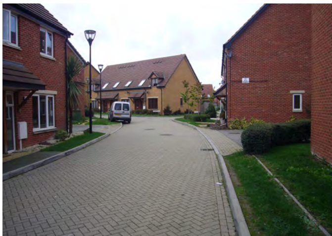
Level surface streets frequently include highway verges. In this example it would have been better for the soft verge to have been a continuation of the block paving to make a wider carriageway.
