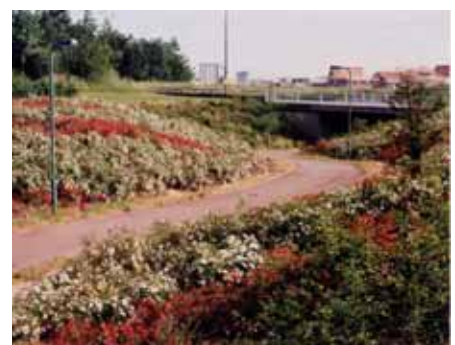
The existing Redway network will be complemented by new Redways throughout the site - however to enhance public safety they will be integrated into the urban form rather than segregated as in this example
