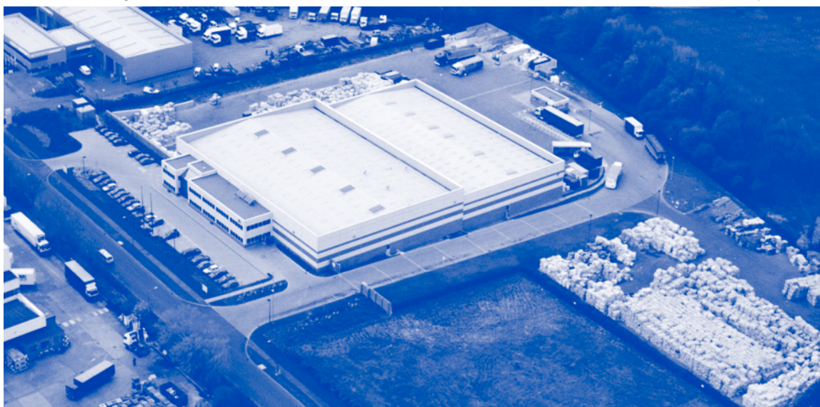
Materials Recycling Facility (MRF) in Old Wolverton
