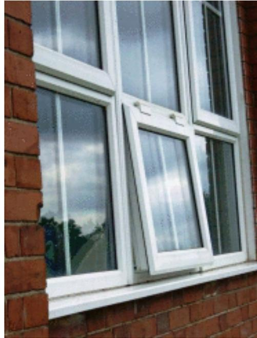
Picture 3.7 Ungainly plastic windows with protruding casements, mitred joints and polythene finish are a conspicuous and discordant alternative to timber. Their medium to long term benefits are increasingly called into question
