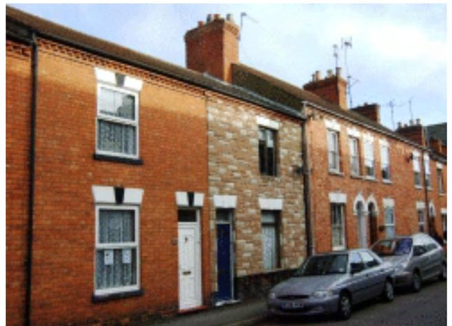
Picture 3.8 Stone cladding is harmful to the appearance and fabric of individual terraces. It causes the eye to be drawn to a discordant alteration at the expense of authentic character
