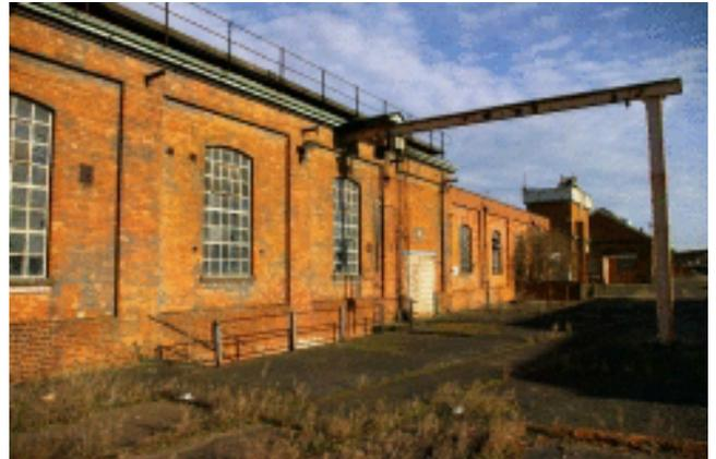
Picture 2.36 Iron windows set in pier and panel construction
