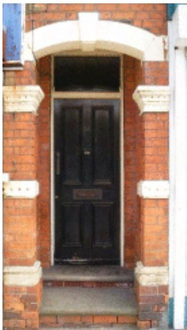
Picture 2.48 Surviving panelled door on The Square (east side), the door is further distinguished by a large transom light and stone detailing (now painted) on the porch entrance
