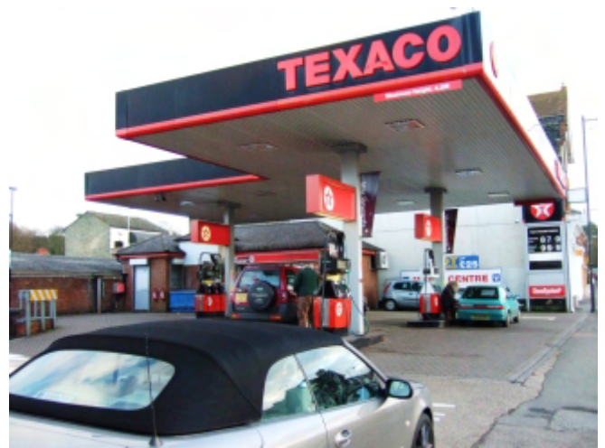
Picture 40 The petrol station canopy
