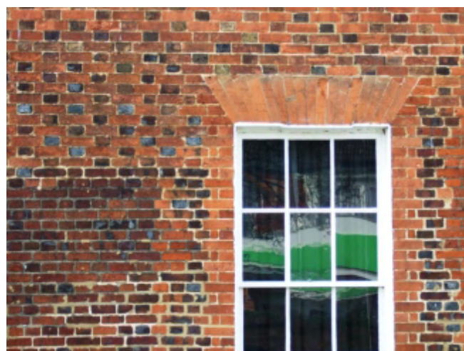
Picture 53 Patterned brickwork and a rubbed brick flat 'arch' above a window on Shelton House
