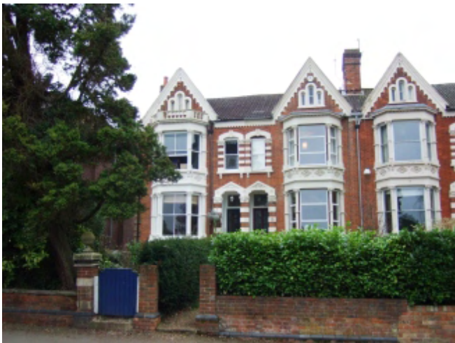
Picture 22 Station Road, numbers 6 - 8
