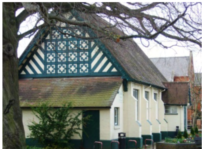
Picture 36 The Institute building, High Street. From an oblique angle the architectural reference to England's great aisled (and buttressed) barns is evident.
