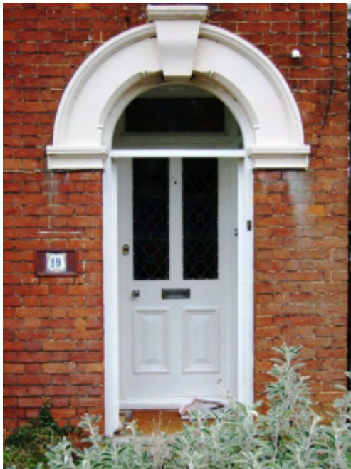
Picture 1 elegantly composed doorways add to the special character of the conservation area
