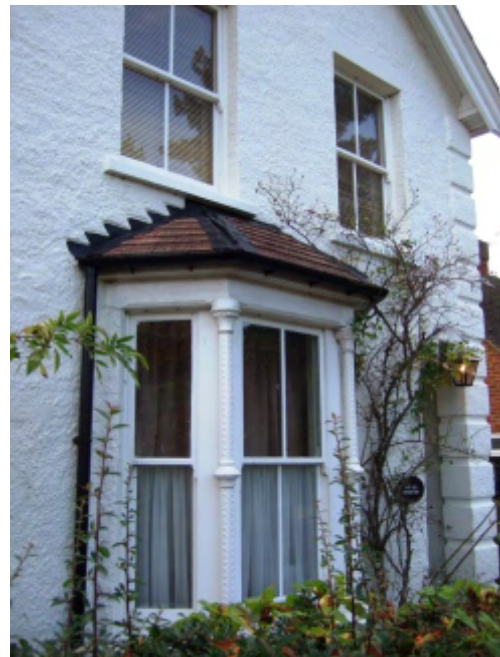
Picture 55 The Old Presbytery survives well, although the painted roughcast is unlikely to have been part of the original finish
