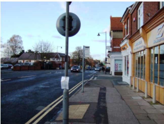
Picture 63 Worn paving, service trenches and the predominance of tarmac combine to create a barren environment
