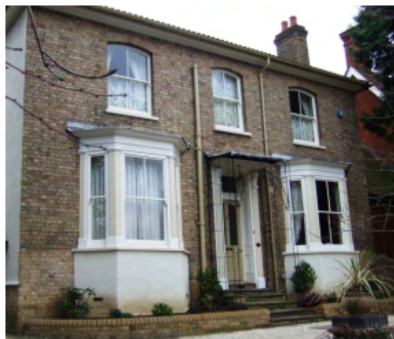
Picture 48 An imposing house on Station Road. Note the lead topped canted bays either side of the front door which itself is set behind ornate open work in wrought iron. The downpipes are in iron.
