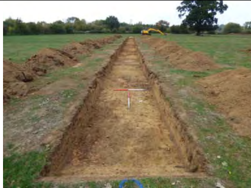
General view of Trench 81, looking west-northwest Fig 127
