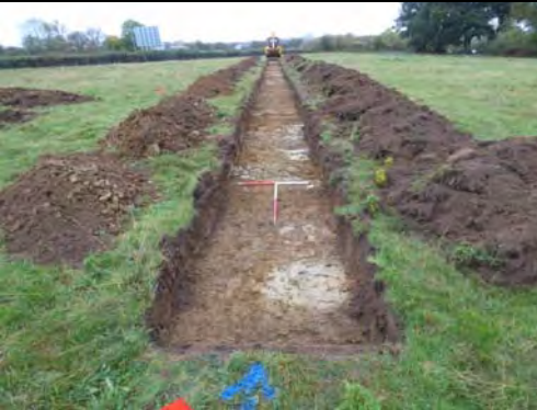
General view of Trench 68, looking west Fig 115
