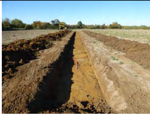
General view of Trench 55, looking west-northwest Fig 104
