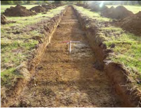
General view of Trench 90, looking east Fig 136
