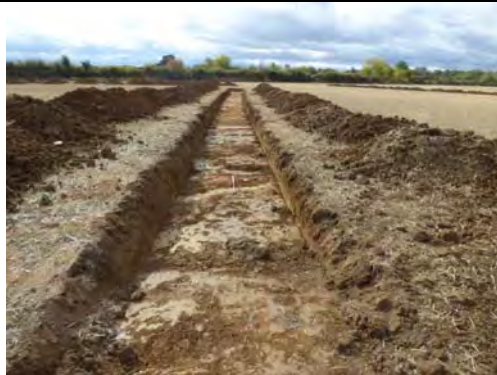
General view of Trench 28, looking south-west Fig 77
