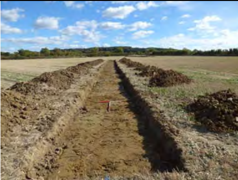
General view of Trench 50, looking west-northwest Fig 99
