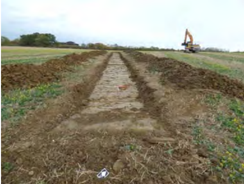
General view of Trench 31, looking northwest Fig 80
