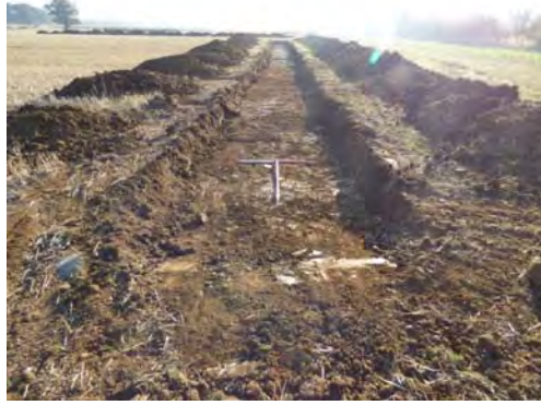
General view of Trench 2, looking east Fig 51
