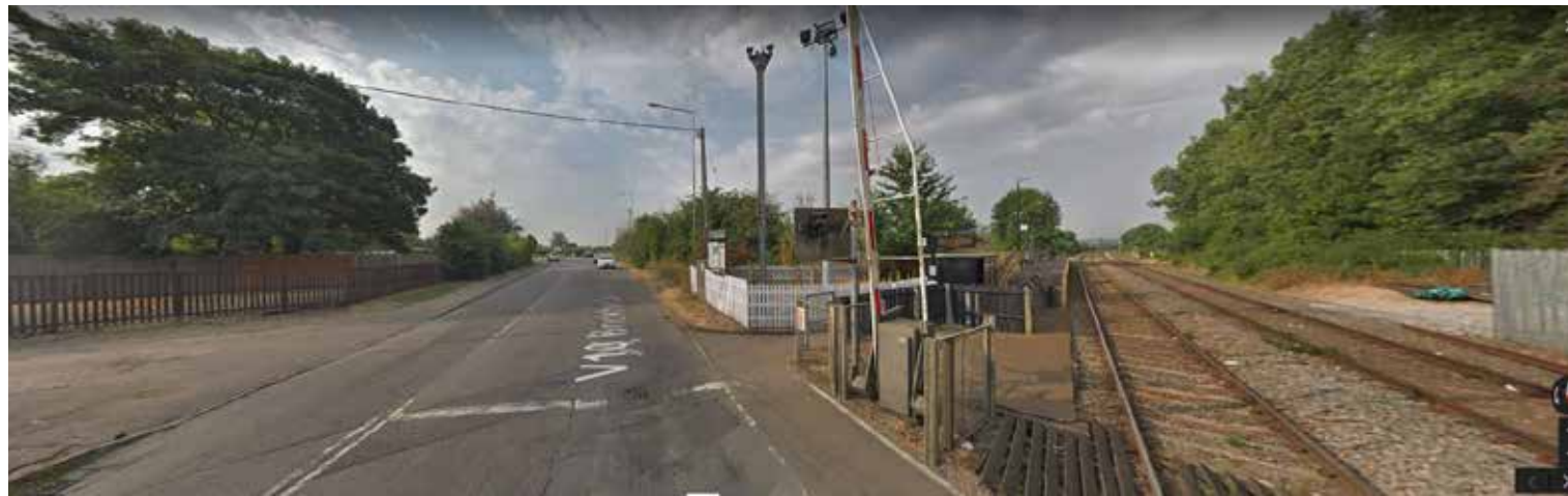
Figure 4.10g The View Looking South along Brickhill Street
