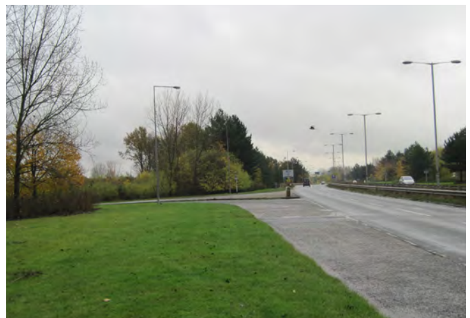
Existing vehicular access to sewage works.
