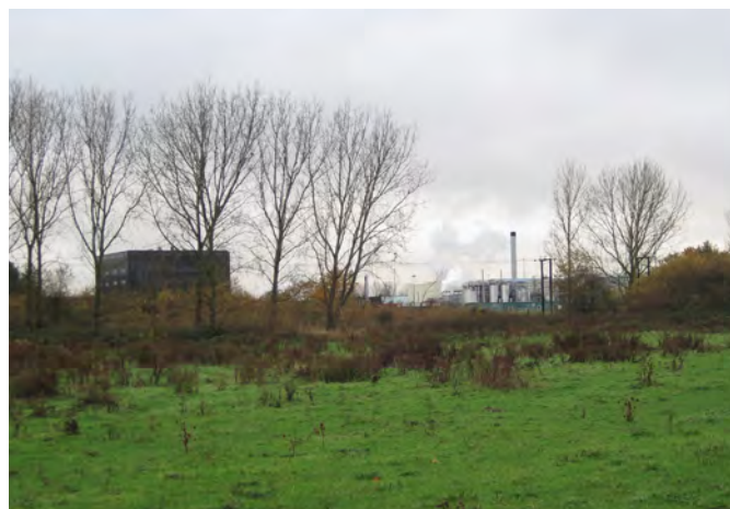
Cotton Valley Sewage Works
