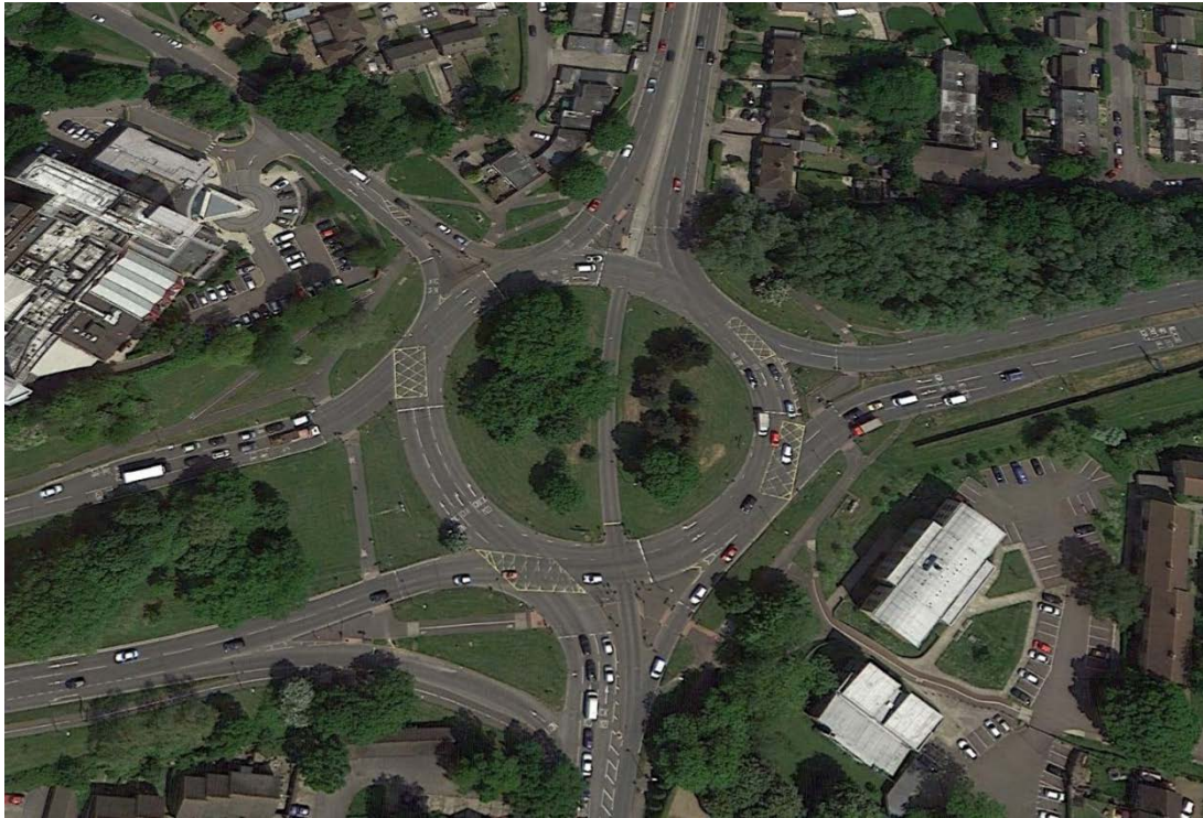
Figure 4-11: 'Hamburger' signalised roundabout junction in Crawley
