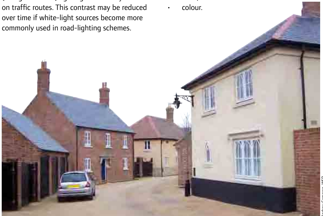
Figure 10.3 Street light mounted on a building.
