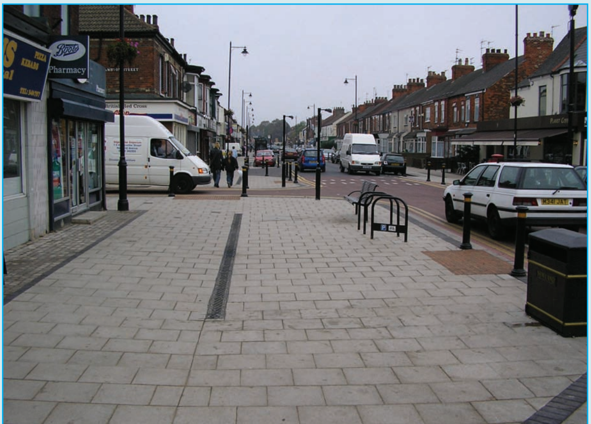
Footways widened significantly by narrowing carriageway
