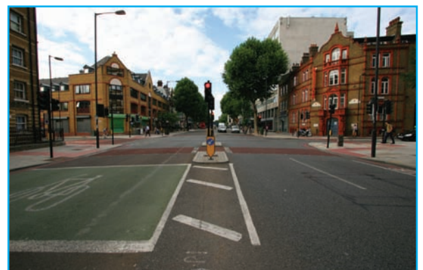
Traffic signal junction with clear and simple pedestrian crossings and advance cycle stop lines. Note lack of guardrailing and buildings close to junction corner, and tight corner radii.
