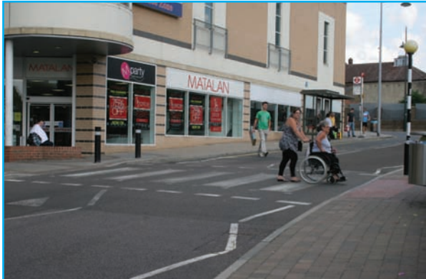
Zebra crossing on raised table.
