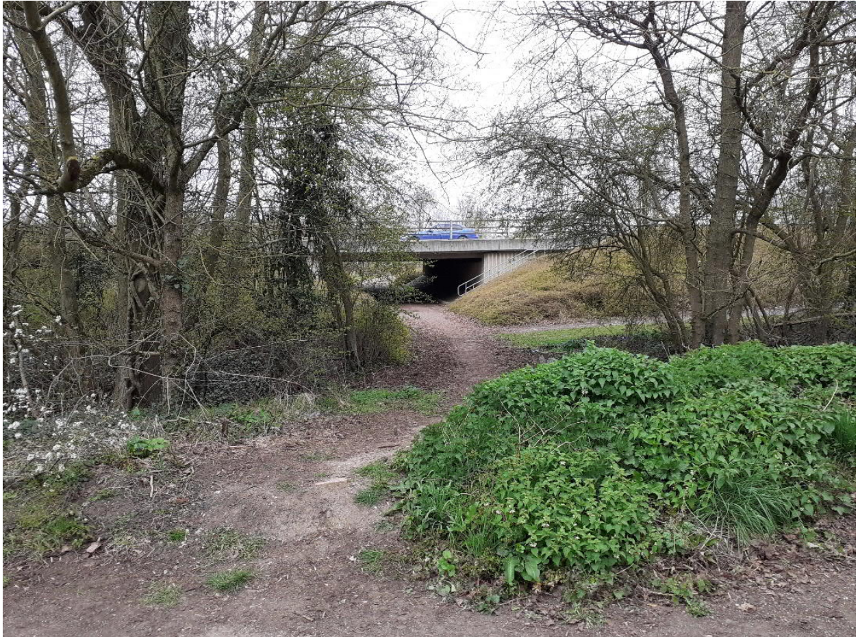
Figure 4-3 - Redway Underpass Access to Old Buckingham Road (Source: WSP Site Visit)
