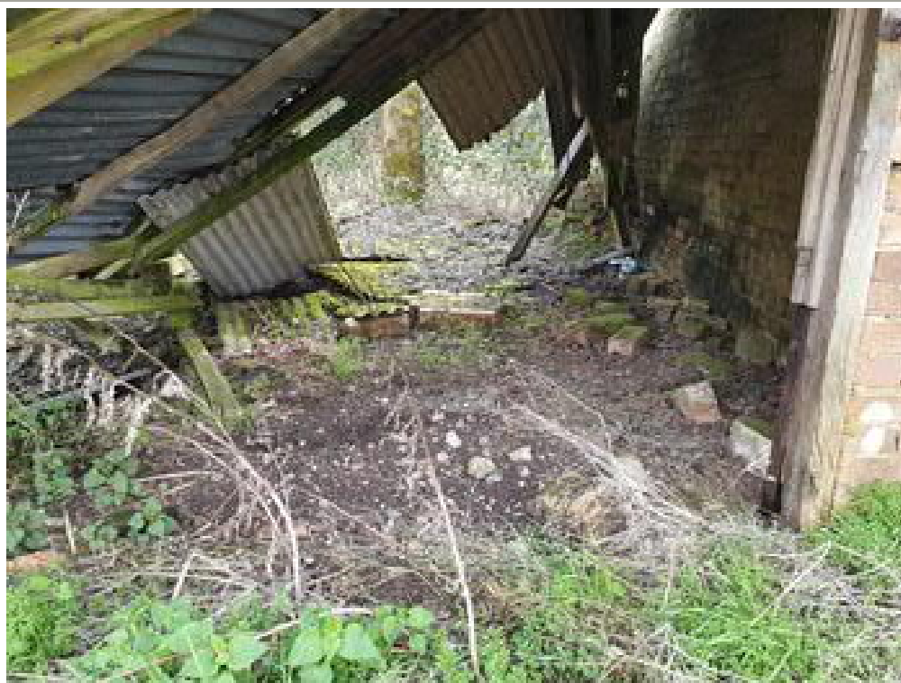
Photo 13 – derelict stable structure and asbestos roof material on the ground
