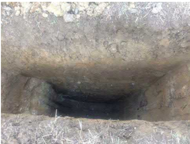
Photo 43: Excavation of trial pit TP04.
