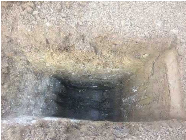
Photo 31: Excavation of trial pit IT06.
