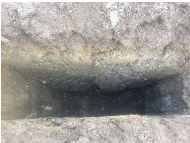
Photo 55: Excavation of trial pit TP10.
