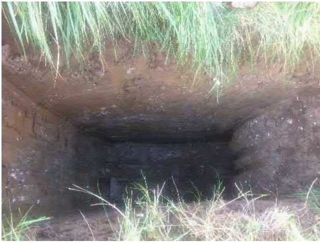
Photo 29: Excavation of trial pit IT05.
