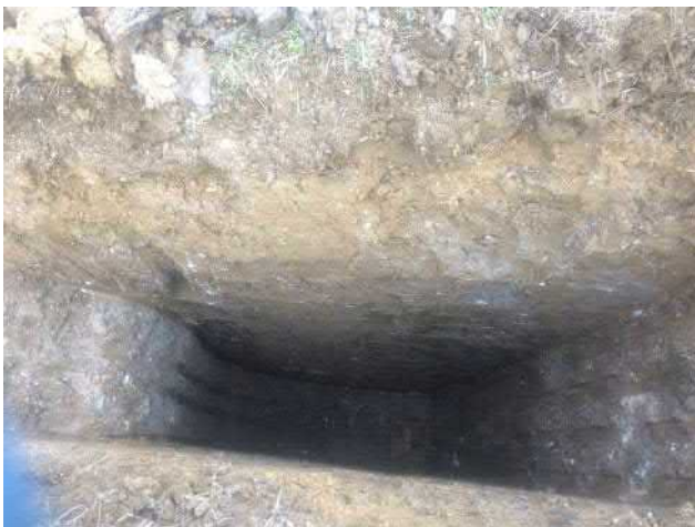
Photo 71: Excavation of trial pit TP18.
