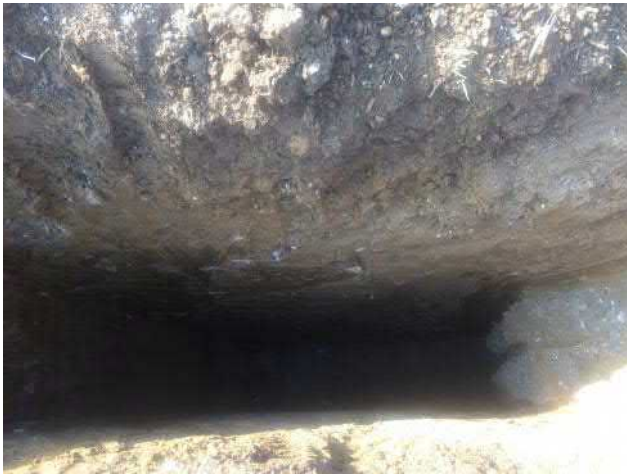
Photo 73: Excavation of trial pit TP19.
