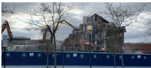
Demolition of Bowback House to make way for 306 apartments - CMK
