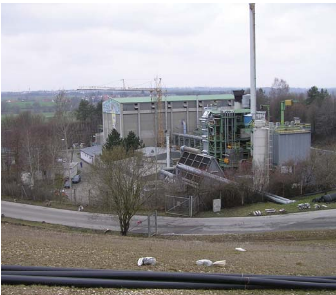
Advanced thermal treatment plant
