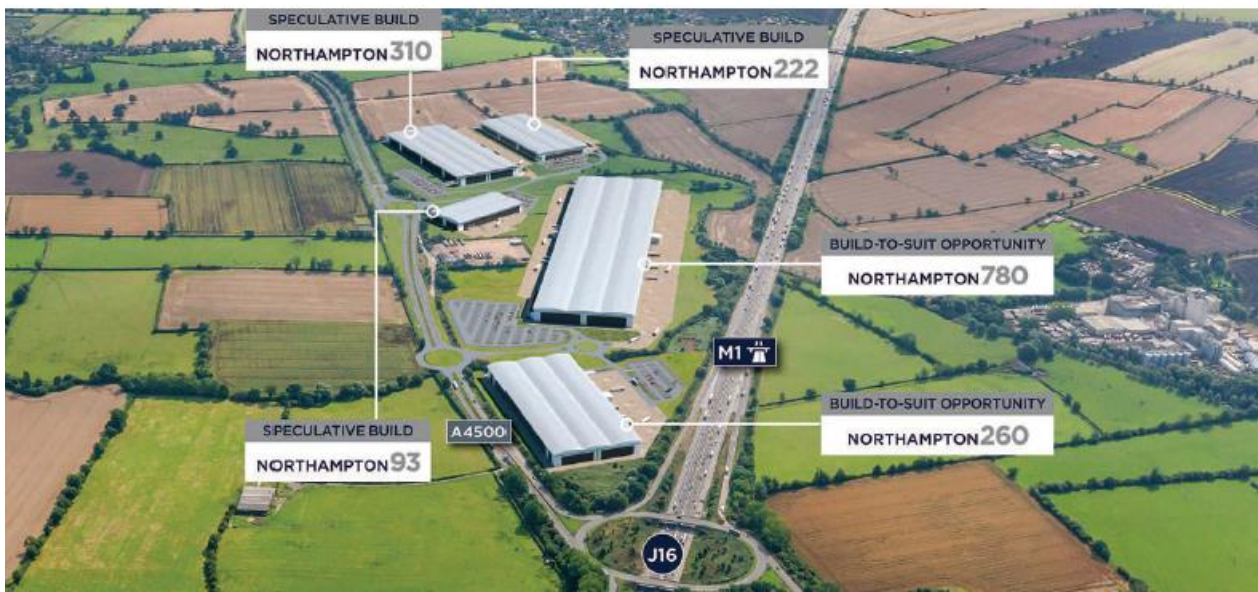
Panattoni Park, Junction 16 of M1, Northamptonshire
