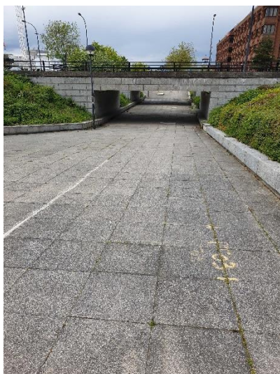
Figure 6-5: Underpass Not Redway
