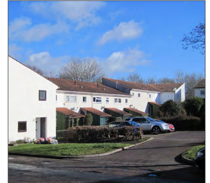
Glovers Lane, Heelands Architect: Henning Larsen
