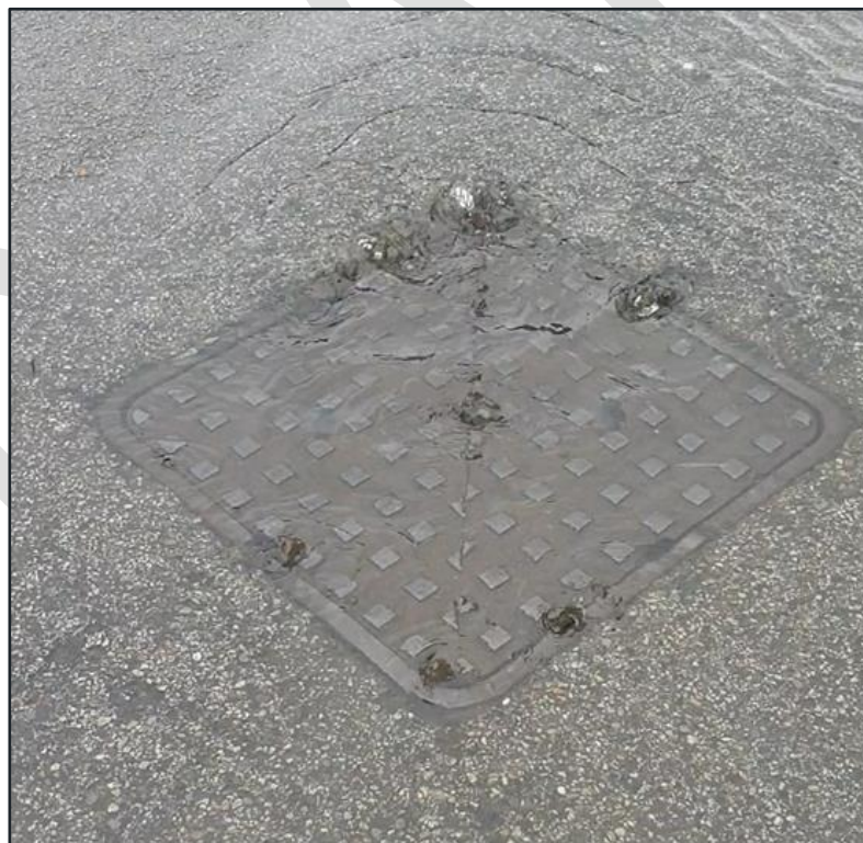
Figure 2-6 – Surcharging manhole on Priory Street, June 2021.
