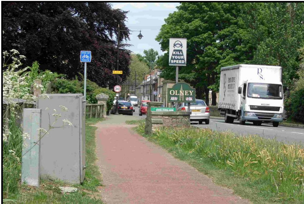
Figure 6: DfT Automatic Traffic Counter (large grey box)
