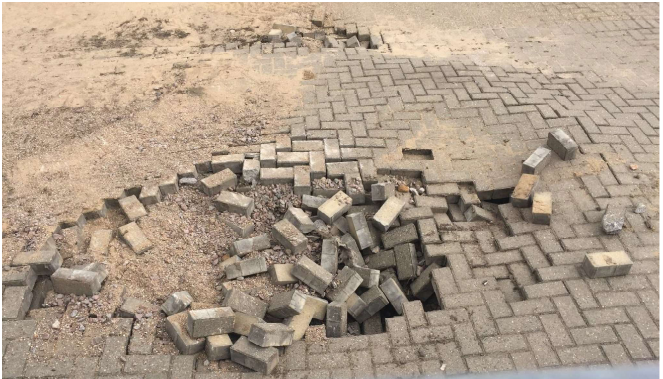
Figure 14 – Pipe Burst Cairngorm Gate
