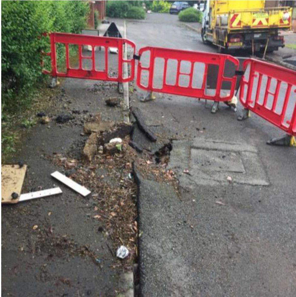
Figure 10 – Damage caused by surface water burst pipe
