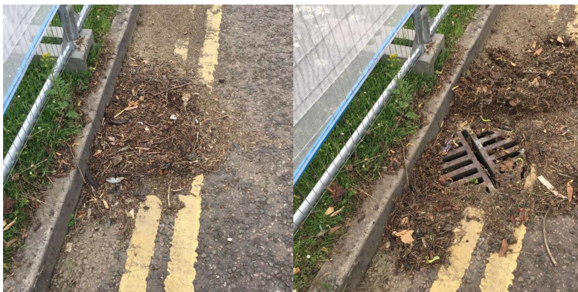
Figure 15 – Road Gully covered in leaf litter and detritus, and uncovered (Cairngorm Gate)
