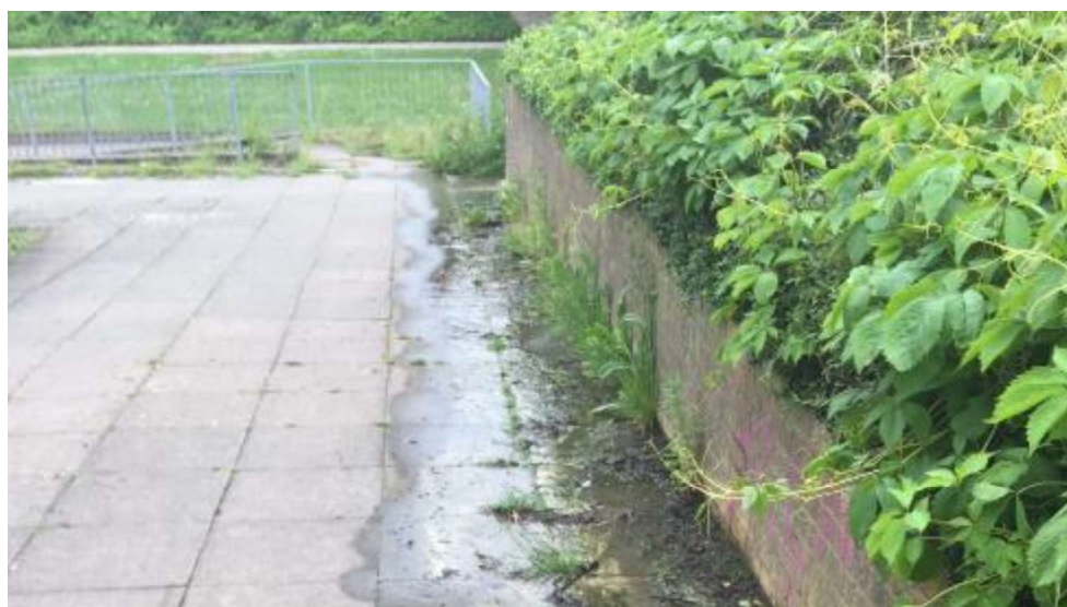
Figure 6 – Evidence of Siltation near to Highway Embankment
