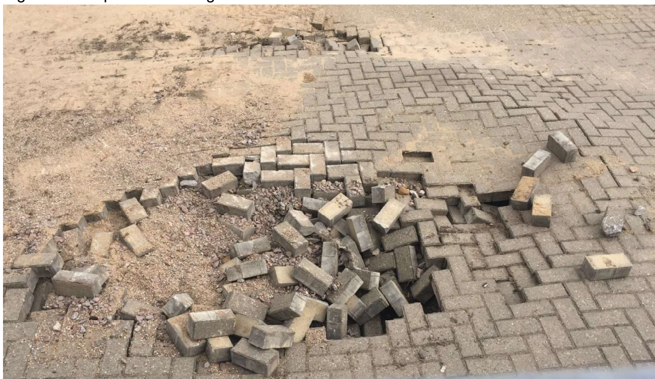
Figure 14 – Pipe Burst Cairngorm Gate
