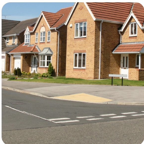
Dropped kerb for pedestrians with tactile paving
