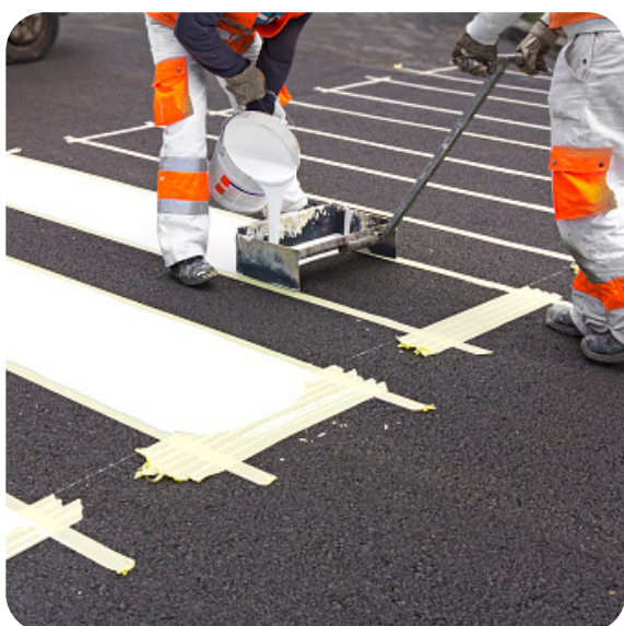
Applying white paint for a Zebra crossing
