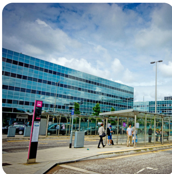
Granite kerbs at Station Square, CMK
