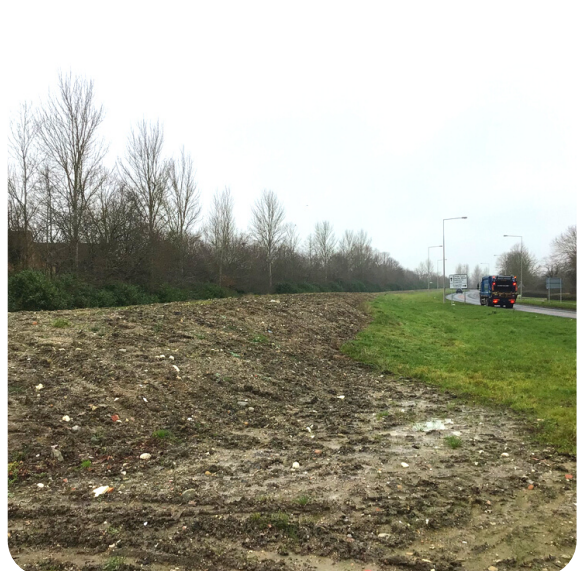
A bund protecting the verge from illegal encampments
