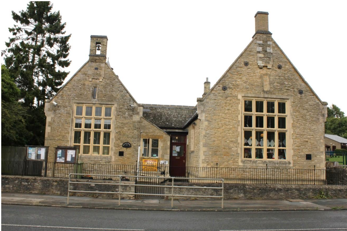
Figure 21: The former village school, now a children's nursery.
