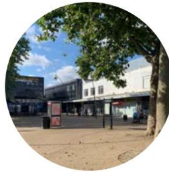
Stanier Square, Queensway is addressed by some poor building facades.
