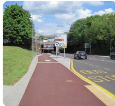
Despite some recent interventions such as the 'Fixing the Links' scheme shown above, provision for cyclists and pedestrians is limited in Central Bletchley.
