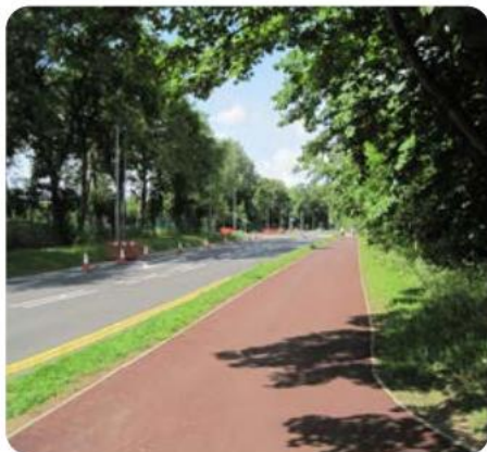
There is currently limited provision for Redways in Central Bletchley with a few exceptions such as along Sherwood Drive to Bletchley Park.
