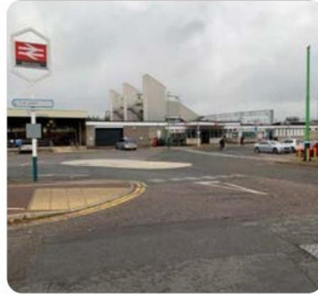
Poor quality western train station entrance.
