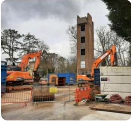
Former fire station: site clearance and remediation in preparation for redevelopment.
