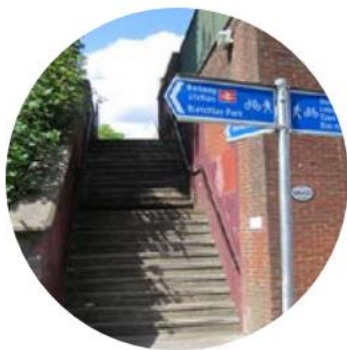
Poor quality pedestrian routes. Including those to the existing Rail Station.
