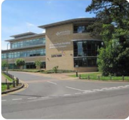
The Andrew Peck building is part of Milton Keynes College located to the west of the CBUDF area. It will be transformed into the new Institute of Technology.
