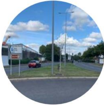
Car dominated streets particularly at the Brunel Roundabout and along Saxon Street.
