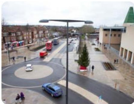
Frideswide Square - Gateway to Oxford, illustrates how an improved public realm can provide a sense of arrival.
