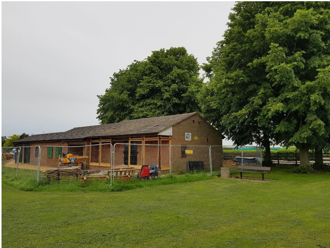
Refurbishment of the Pavilion on the Recreation Ground
