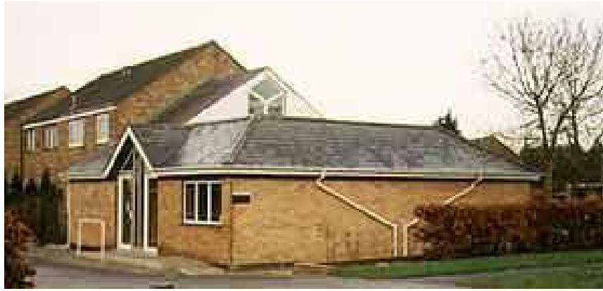
The new Doctors Surgery – at the Western Drive junction with Castlethorpe Rd
