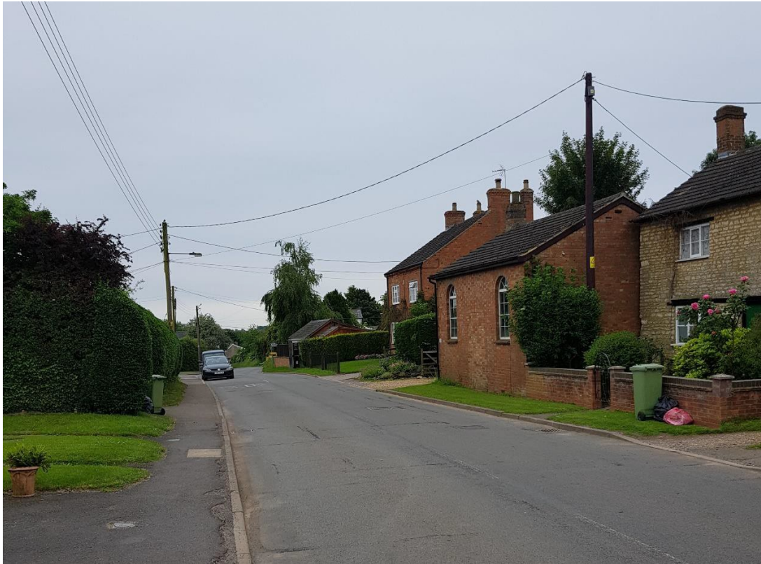
View down from Long Street to Hanslope
